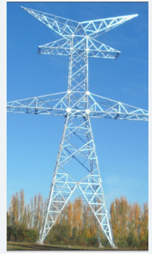
500 kV Danubio Tower 64m tall and 65t
