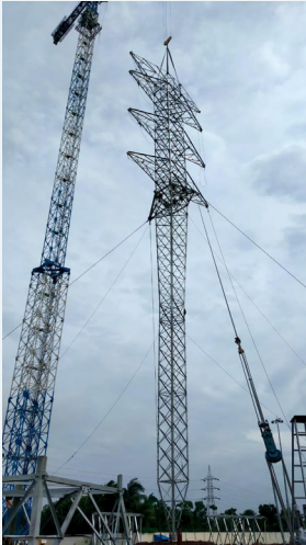
330 kV Guyed Suspension 56m tall and 16t
