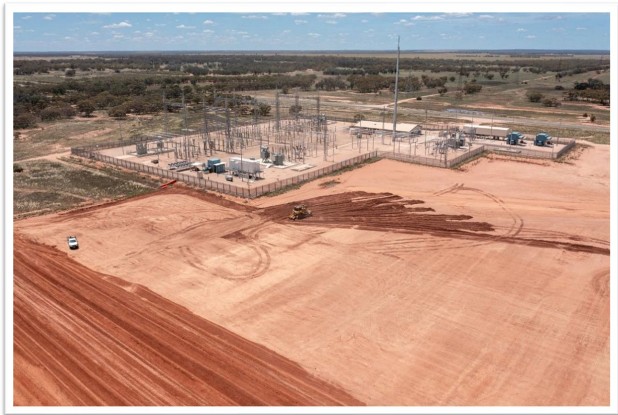
Image 2: Aerial view of the existing Buronga Substation and construction works
