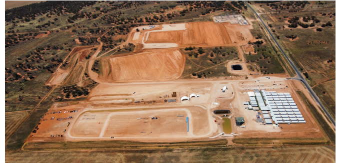
Existing Buronga Substation and extension construction works
