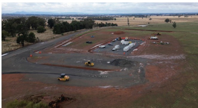
Establishing the road access point at the Lockhart Camp
