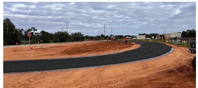
Improving road access points to main construction activities and water sources
