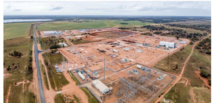
Existing Buronga Substation and extension construction works
