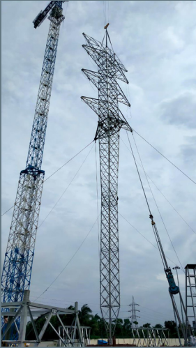
330 kV Guyed Suspension 56m tall and 16t
