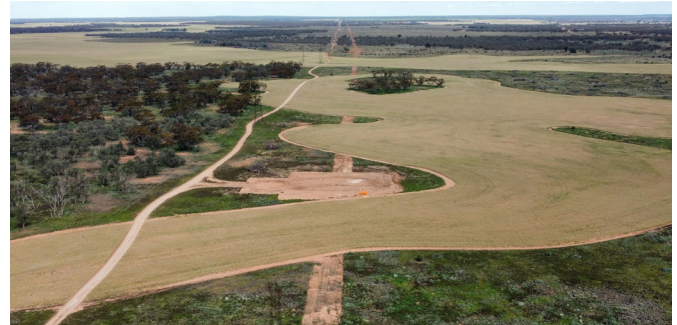
Foundation pads ready to commence tower assembly
